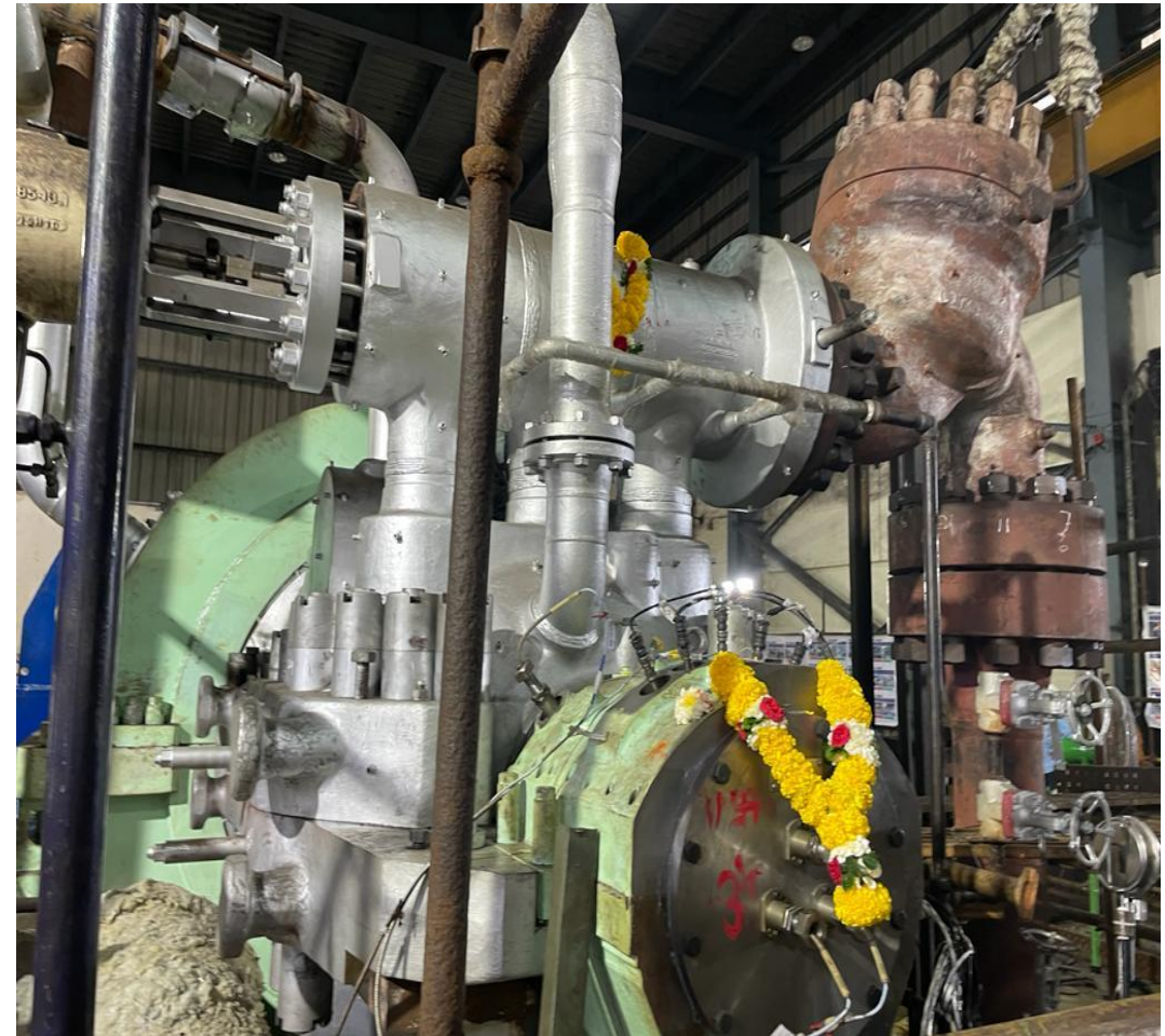
Waste heat recovery Power Plant – Turbine Upgradation
